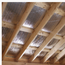
Metal Roof With Insulation
