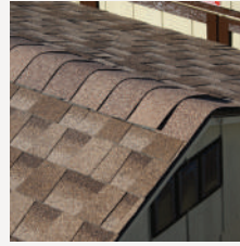
Shingle over Ridge Vent
